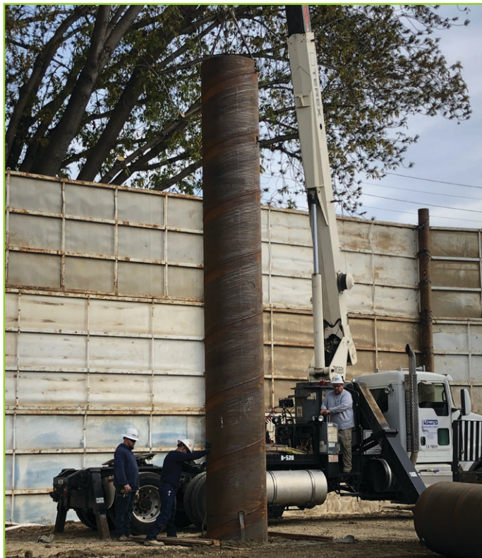
Installation of conductor.
