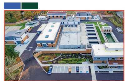
LAKE OSWEGO WATER TREATMENT PLANT UPGRADES & EXPANSION
