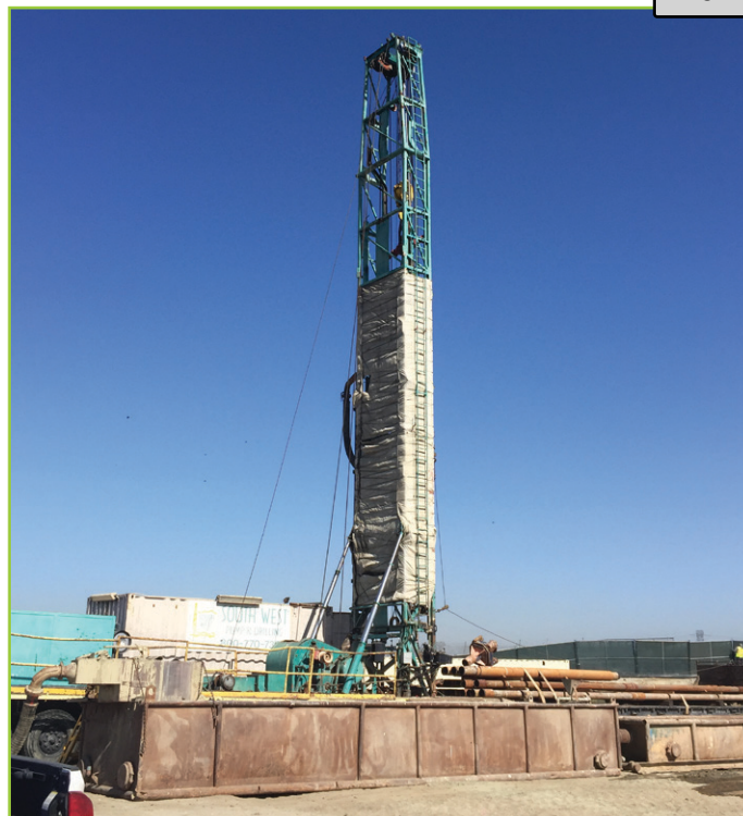
Pilot borehole drilling for CDA-II-12
