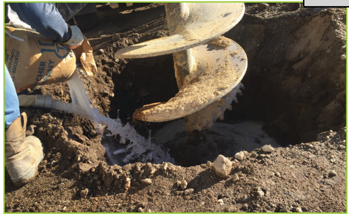
Auger drilling for the conductor casing placement
