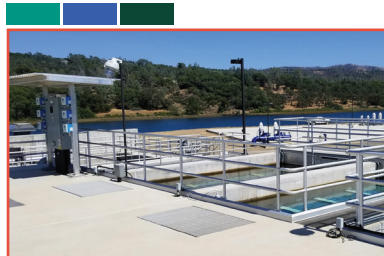
MINERS RANCH WATER TREATMENT PLANT IMPROVEMENTS PROJECT
