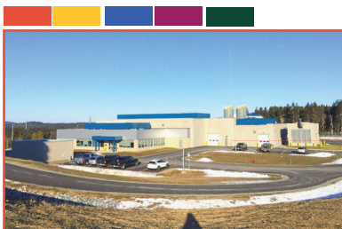
SAINT JOHN WATER TREATMENT PLANT
