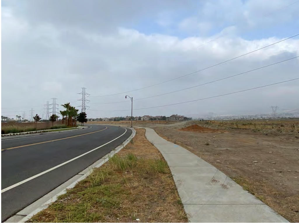
LOOKING WEST DOWN KNOX AVE. NEAR THE SUBJECT'S SOUTHEAST CORNER
