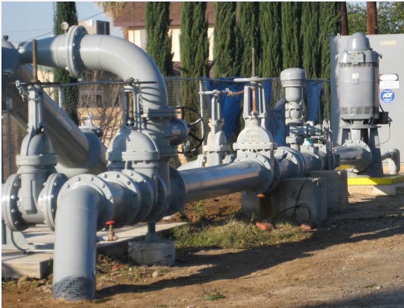
Existing Groundwater Extraction Well.
