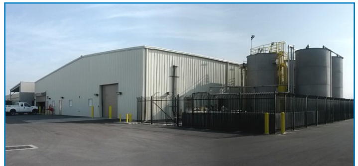
Existing Water Treatment System in Rialto.
