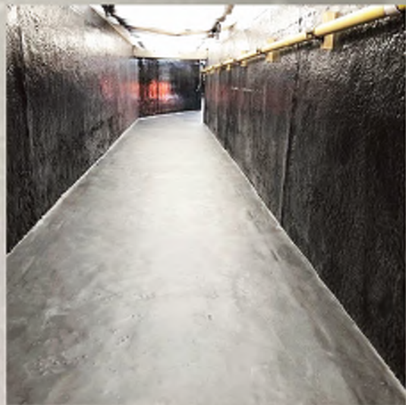
Elastomeric Polyurethane Coating on Concrete
