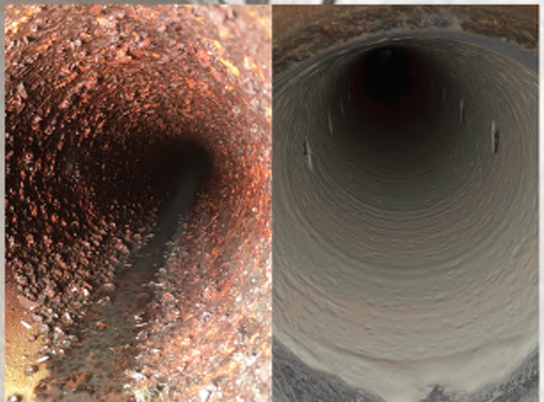
Blast and coatings of Piping Interior
