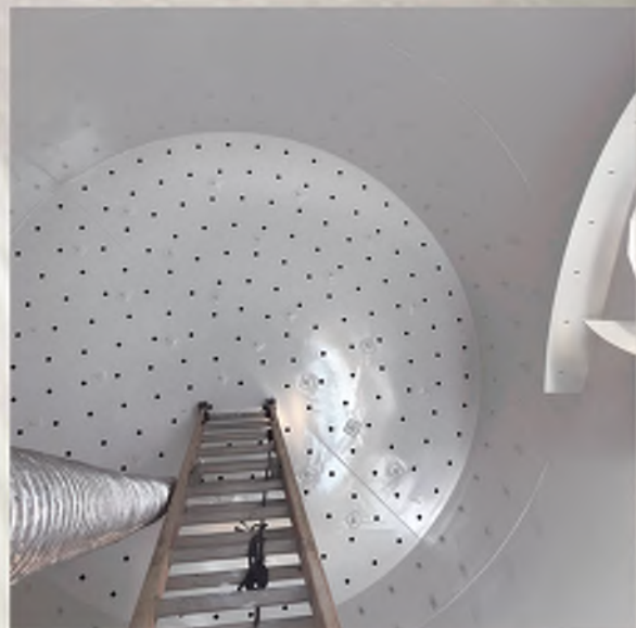
Epoxy Coating on Steel
