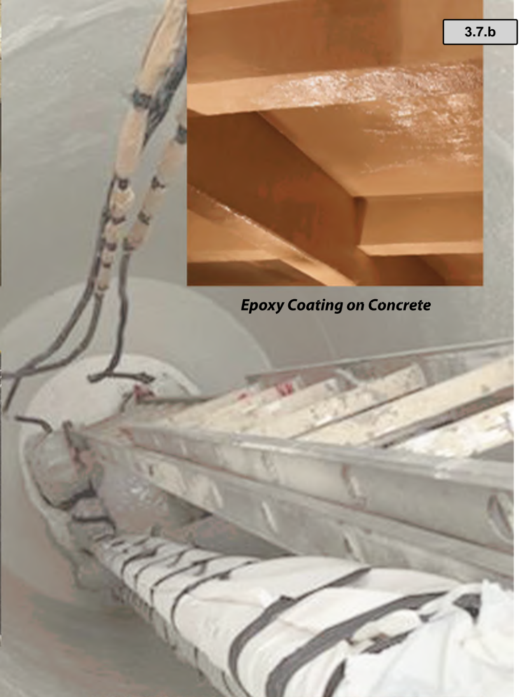
Elastomeric Polyurethane Coating on Concrete
