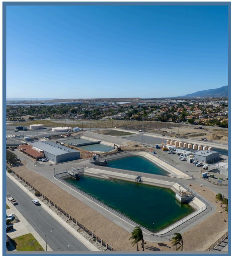
Pictured: Oliver P. Roemer Water Filtration Facility
