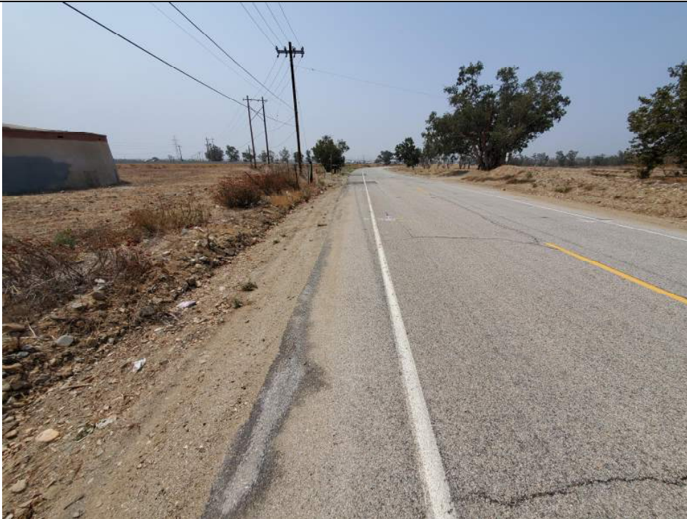
Photo 1. North side of Project alignment; looking southwest along Lytle Creek Road, where the proposed 18-inch CML&C transmission water main would connect to an existing 18-inch transmission main at Lytle Creek Road.
