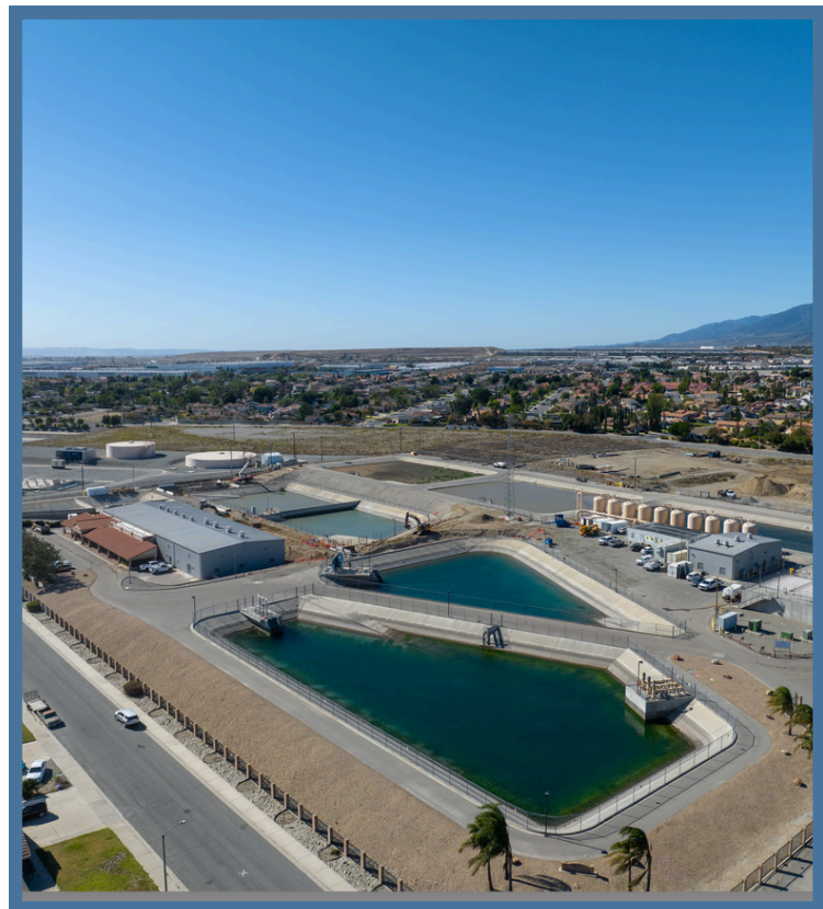
Pictured: Oliver P. Roemer Water Filtration Facility
