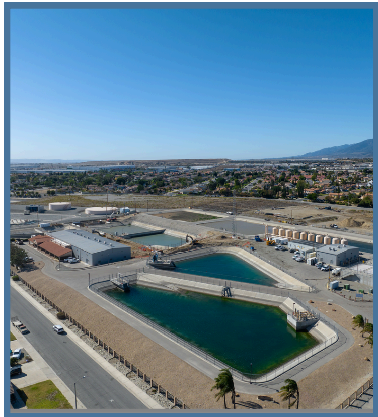
En la foto: Oliver P. Roemer Water Filtration Facility
